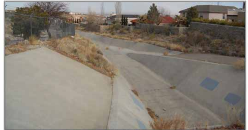
Many arroyos in urban areas have been hardened, channelized, and fenced off. Rather than serving as habitat and a public amenity, they are relegated to the rears of houses and seem to be nothing more than engineered stormwater conveyance infrastructure.
